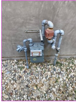
Gas meter condition
