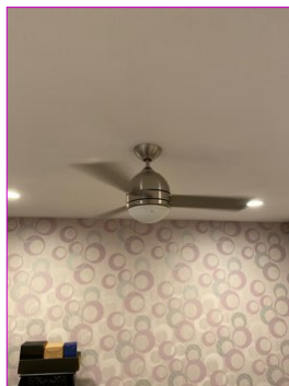
Ceiling fan condition
