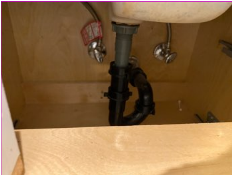
Plumbing under left side sink
