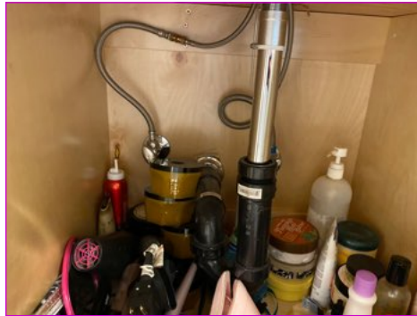
Plumbing under sink on right
