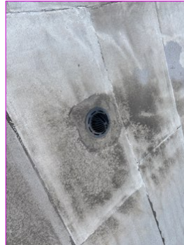
In roof drain above the garage
