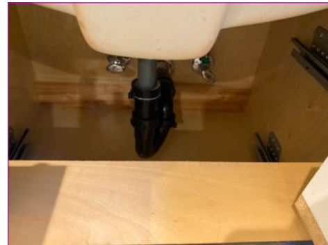
Plumbing under right side sink
