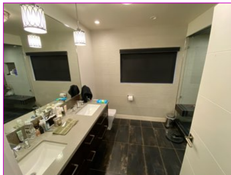
Master bathroom condition
