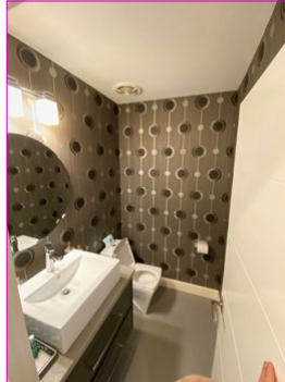
Entry bathroom condition
